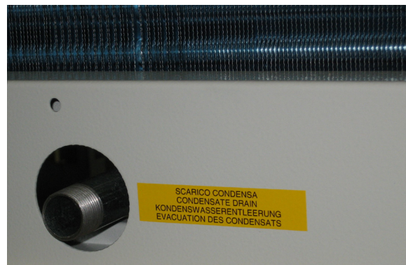
Fig. 10 Connection to the condensate collection tray
